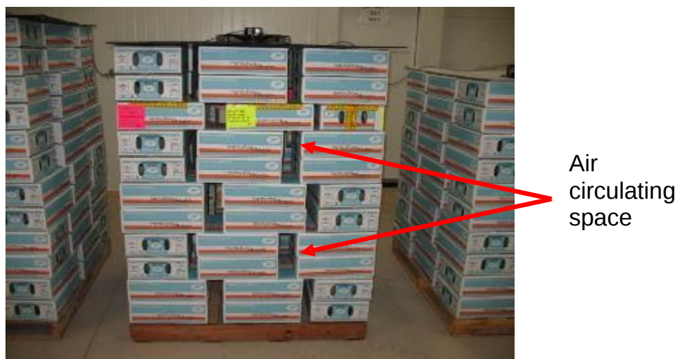
Figure 1: Instructions for arranging packages in the cold room
